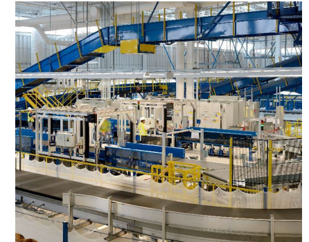
Canada Post Processing Facility, BC
