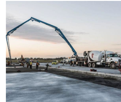
YVR South Airport Cargo Project
