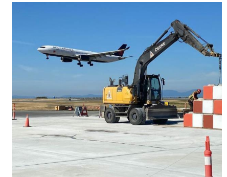
YVR South Airfield Pavement Rehab
