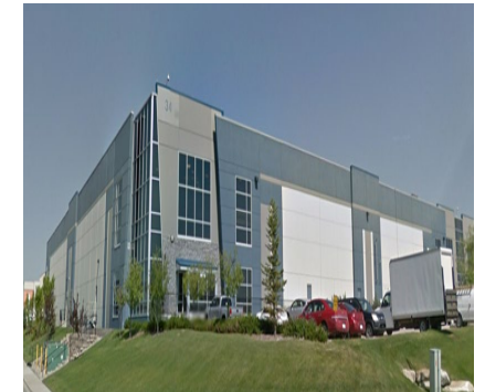
Rogers Data Center
