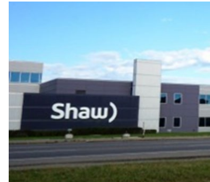
Shaw Campus Data Center
